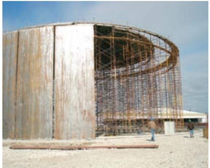
Stages of construction of the 5 million gallon reinforced concrete storage tank. Above, erecting precast panels.
