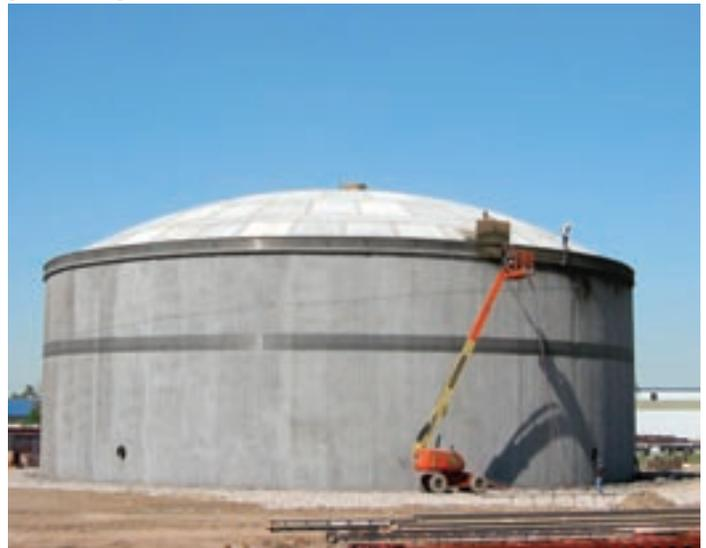
Applying the 'post-tension' wiring to provide steel reinforcement for the tank.
